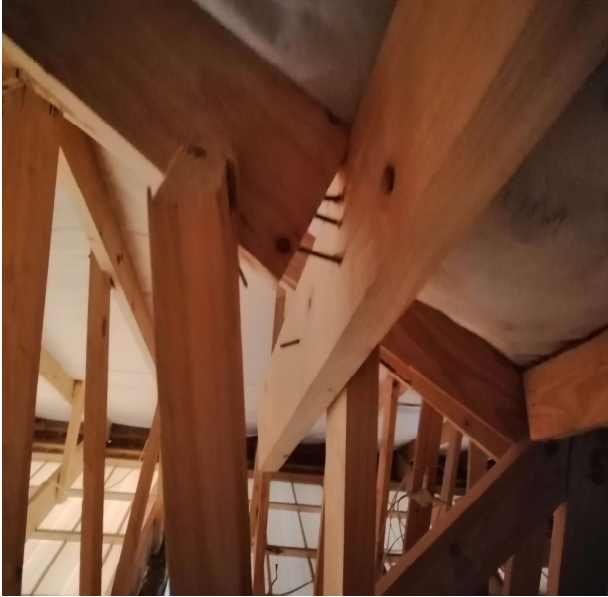
Fig 6- Loose connection
