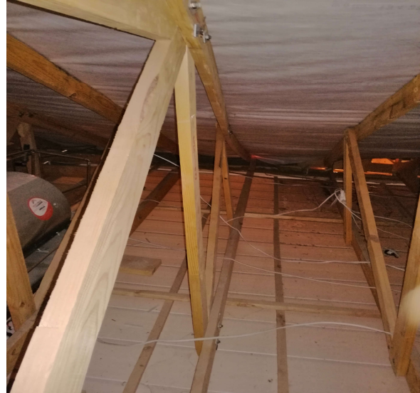
Fig 5 – Buckled Trusses
