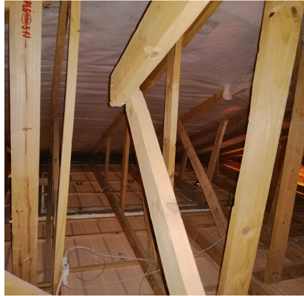
Fig 7 Truncated truss
