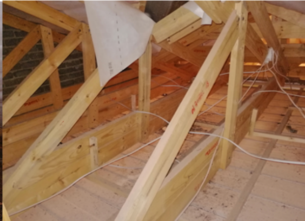
Fig 9- Stiffened bottom sections
