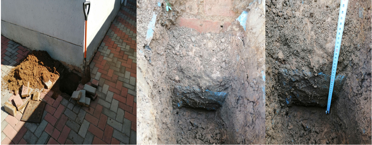
Fig 10- Exposing foundation Fig 11- Exposed footing Fig 12- Footing thickness
