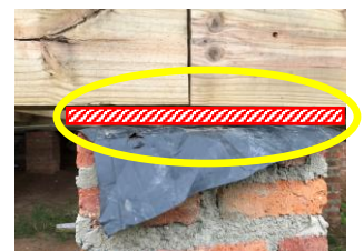
No support or fixing
