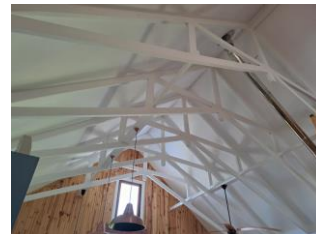
Roof truss completed
