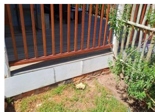
Exterior with no aprons
