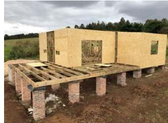
Cladding in progress
