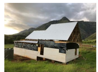
Isolation and Cladding
