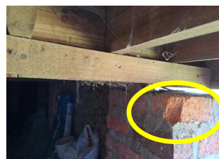
Damaged bricks
