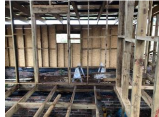
Exposed timber sections
