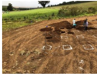
Excavations for Bases
