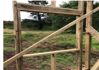
Exterior timber panel
