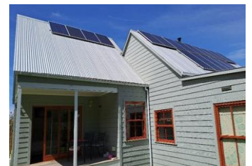
Completed roof with sheeting
