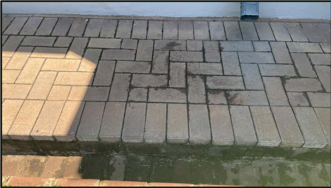
Figure 5: Showing the brick paving around the house.
