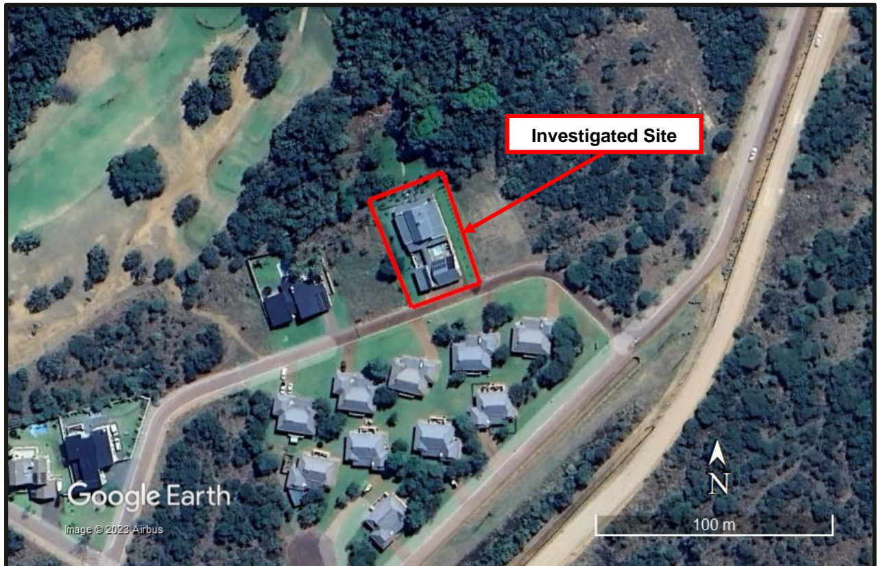
Figure 1: Showing the investigated house (red outline) in Thorny Bush Estate, Mokopane.
