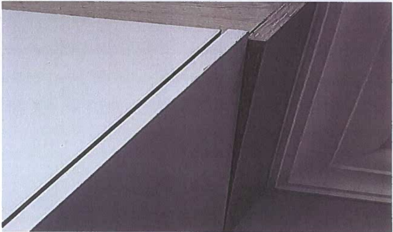
Plate 13 supplements plate 11 and 12 but showing misalignment of the build in closets attributed to the foundation movement.
