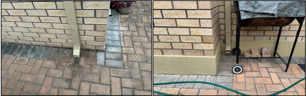
Figure 6: Showing the gutters around the investigated house.
