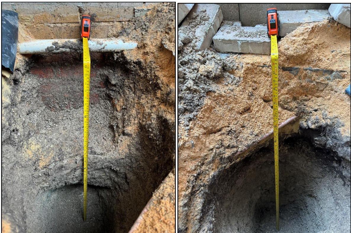
Figure 5: Showing test pit HB1.
