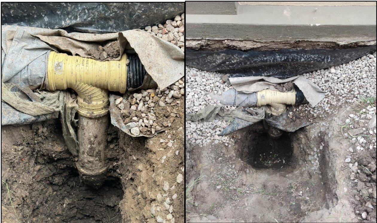
Figure 7: Showing the stormwater pipe in the garden area.
