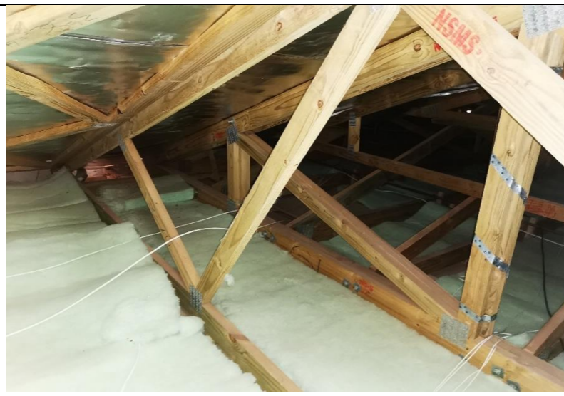
Photo 5: Timber roof trusses
