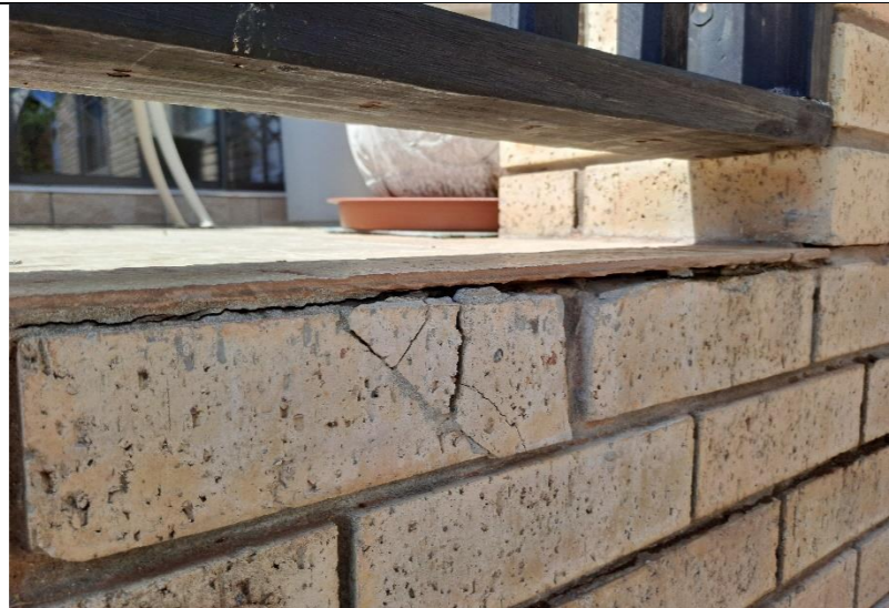
Photo 4: Delamination of floor tiles.
