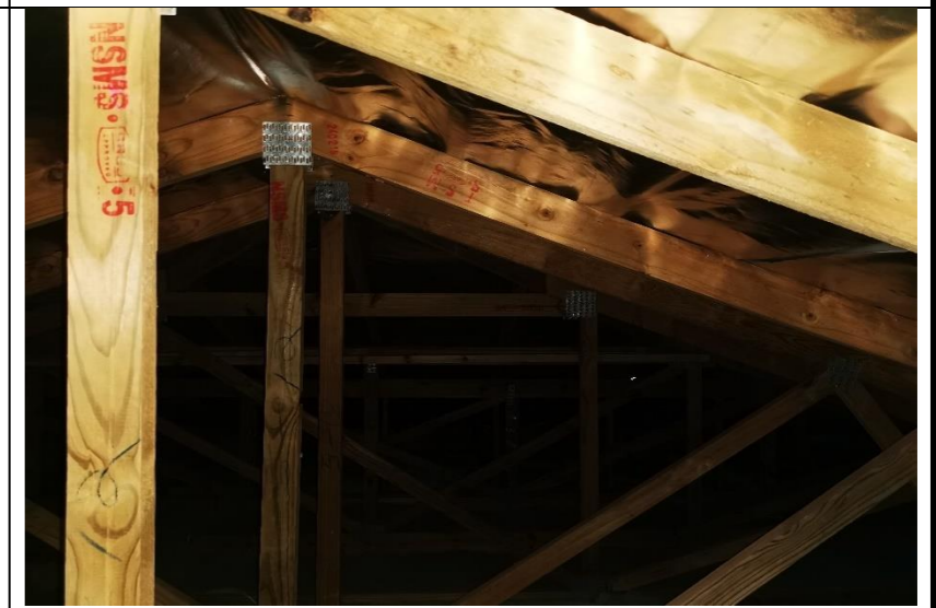
Photo 6: Timber roof trusses
