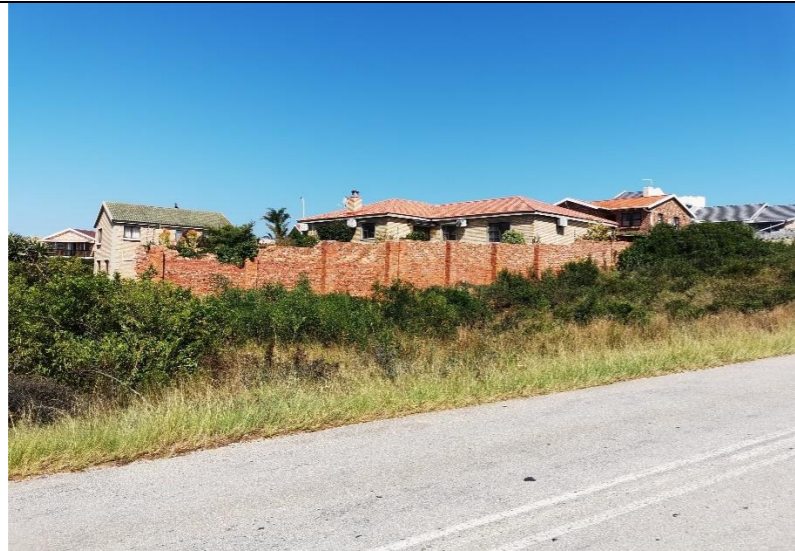
Photo 1: General site view.
