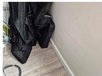
Pic 11: Rising damp on internal wall.
